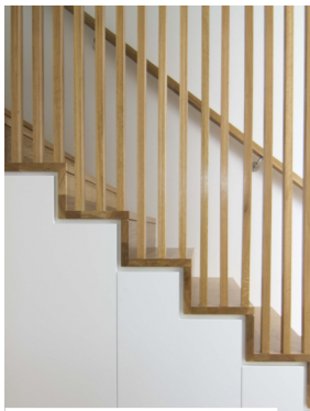
A seamless detail to the staircase and balustrade junction. Concealed storage below stairs to maximise use of space.
